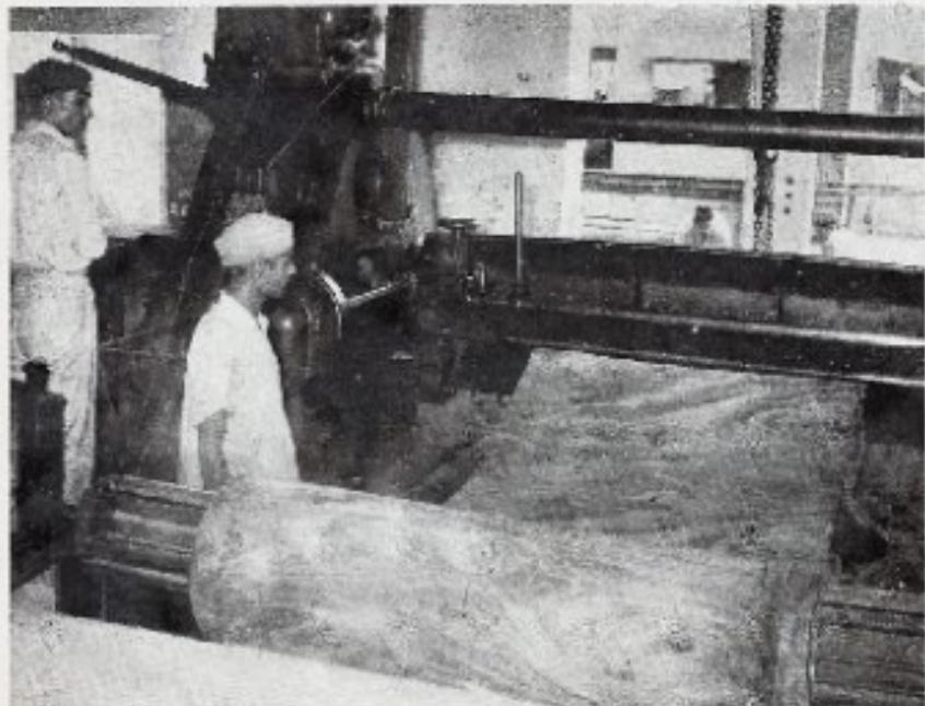
VEENEER PEELING LATHE
