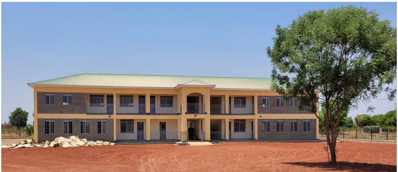
Newly constructed education Center at Loreto Rumbek.
